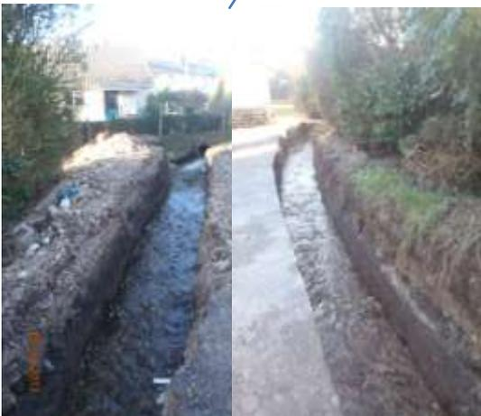
Flooding to the rear of Brooklands resulting from channel behind property being overwhelmed when flows are backed up from highway culvert. Flood relief channel has been constructed to convey flows around property in high flow conditions which is still to be completed.
