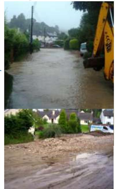
Ditchcourse running adjacent to No.1 Cooks Mead flowing to 450/600 mm culvert passing under Cooksmead into Brooklands. Large accumulation of gravel blocking culvert entrance particularly during high flows. Culvert quickly surcharges and flood waters onto the highway.
