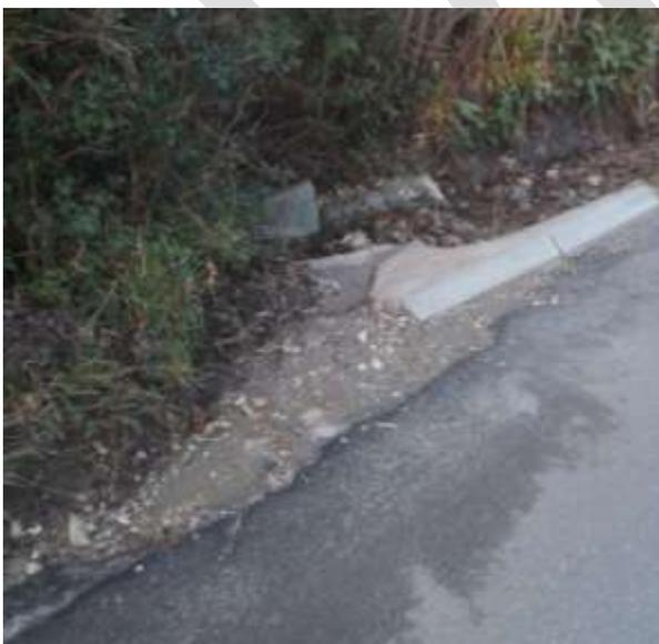
600mm culvert discharging into open ditch at right angles. Downstream channel smaller in capacity than that upstream section. Culvert becomes quickly blocked with large shingle/gravel and floods road.
