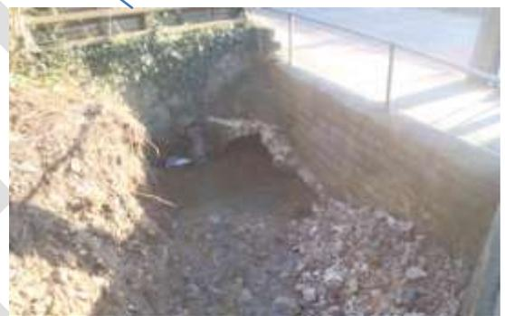
The cross culvert (masonry arch approximately 1mx0.5m) running from the filling station to the village hall surcharges causing flooding of the B3165. Becomes rapidly blocked with shingle/gravel/silt debris and potential for silt trap at this location. Grips were then cut into the verge adjacent to the Village hall car park to allow flood water to re-enter the channel (which was bank fall) and prevent properties adjacent to the highway flooding
