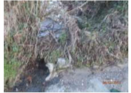
600 mm passing under Lime Kiln Lane/Pounds Lane into ditchcourse running adjacent to No.1 Cooks Mead. Large accumulation of gravel blocking culvert entrance particularly during high flows. Informal silt trap constructed within channel but difficulties gaining access to clear. Formal silt trap could be constructed at this location however culvert immediately upstream suffers blockage and flows onto highway
