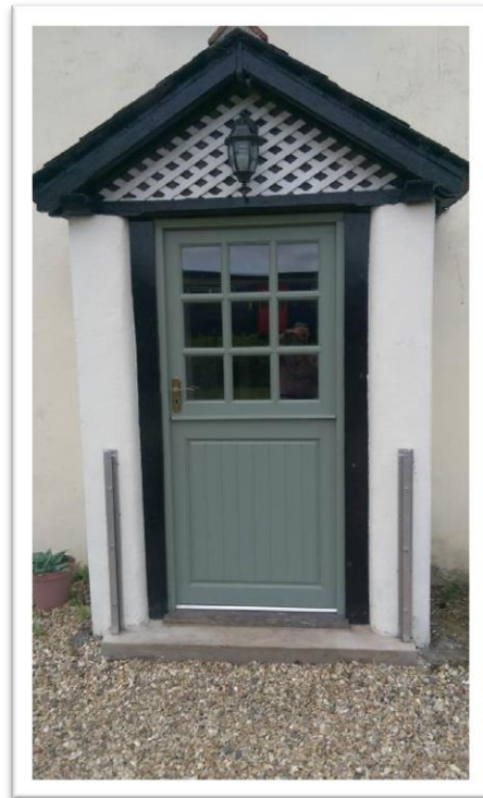
Property front door with slots either side, ready for flood boards to be slotted into place in the event of a flood warning – Umberleigh, North Devon
