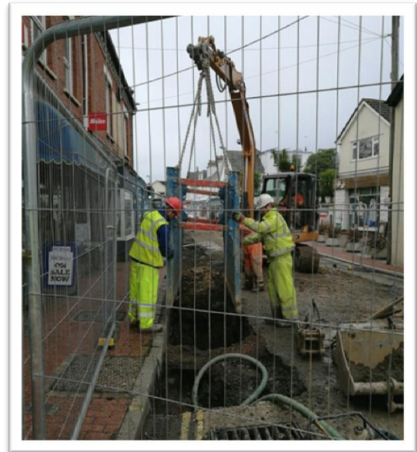
Works to Braunton Flood Defence Scheme – February 2017
